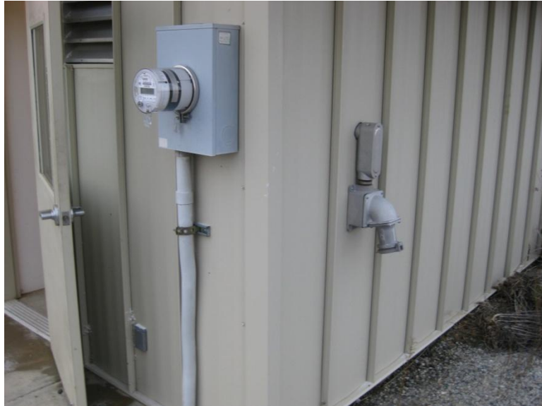
NE OMAK WELL BACKUP POWER CONNECTION
