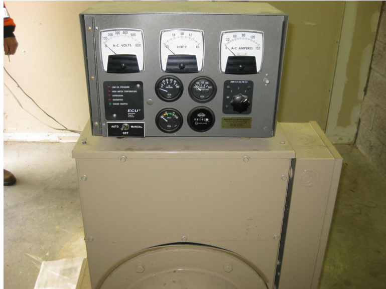
WILDWOOD BOOSTER STATION GENERATOR MONITORING PANEL
