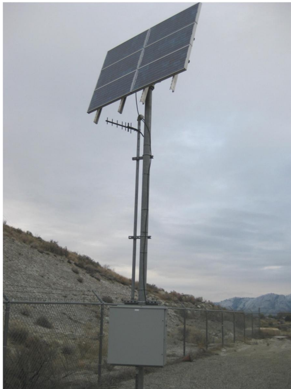
SOLAR PANEL AND TELEMETRY STATION
