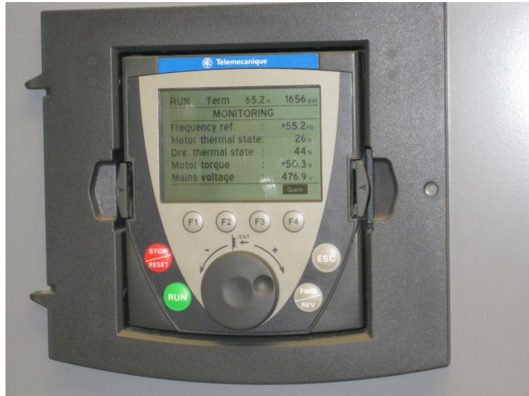
RIVERSIDE BOOSTER STATION VFD CONTROLS
