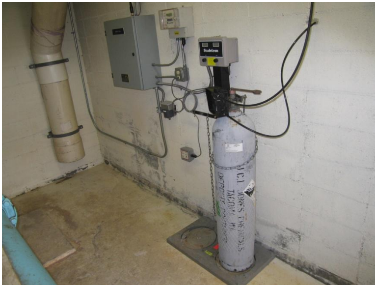
OKOMA WELL CHLORINATION EQUIPMENT
