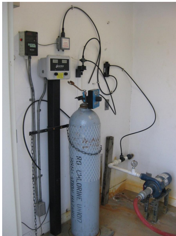
NE OMAK WELL GAS CHLORINATION
