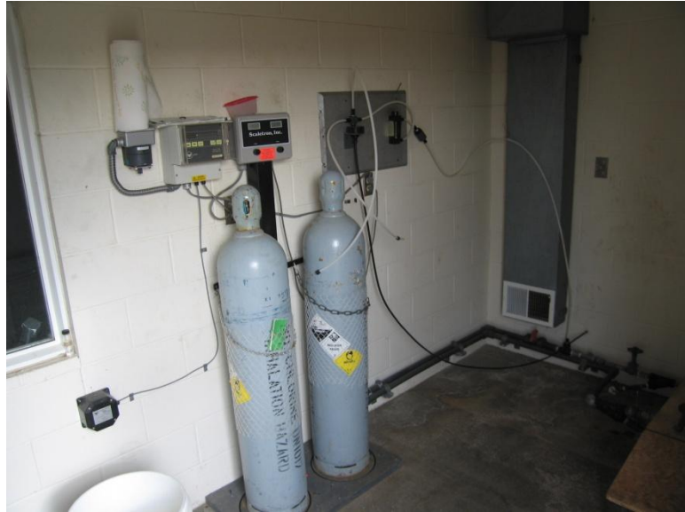
OWP WELL #2 CHLORINATION EQUIPMENT (IN CHLORINATION ROOM)
