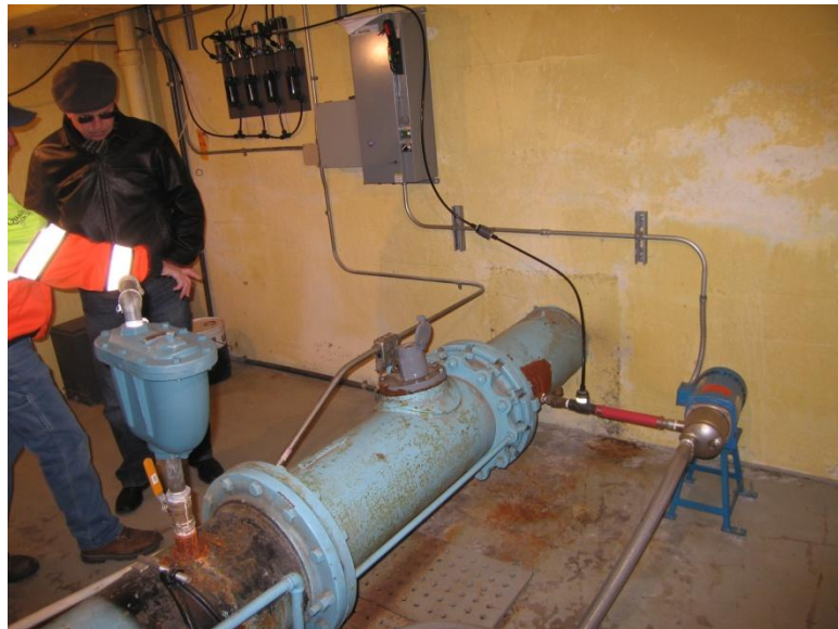
EASTSIDE WELL CHLORINATION EQUIPMENT AND INJECTION POINT
