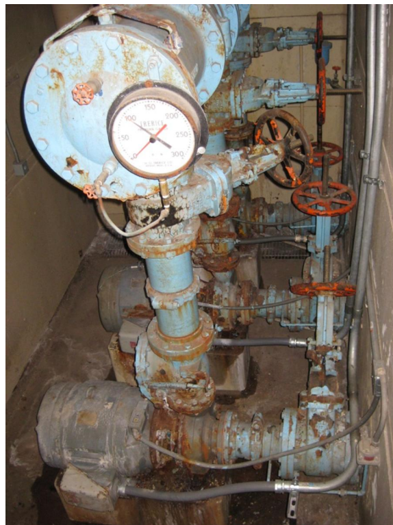
3 BOOSTER PUMPS AT THE ASH STREET BOOSTER STATION
