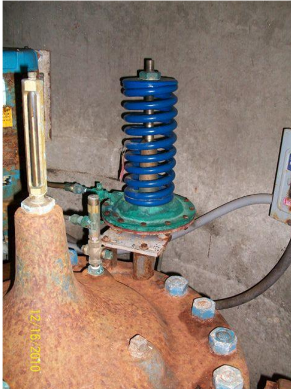
SOUTH HILL RESERVOIR ALTITUDE VALVE
