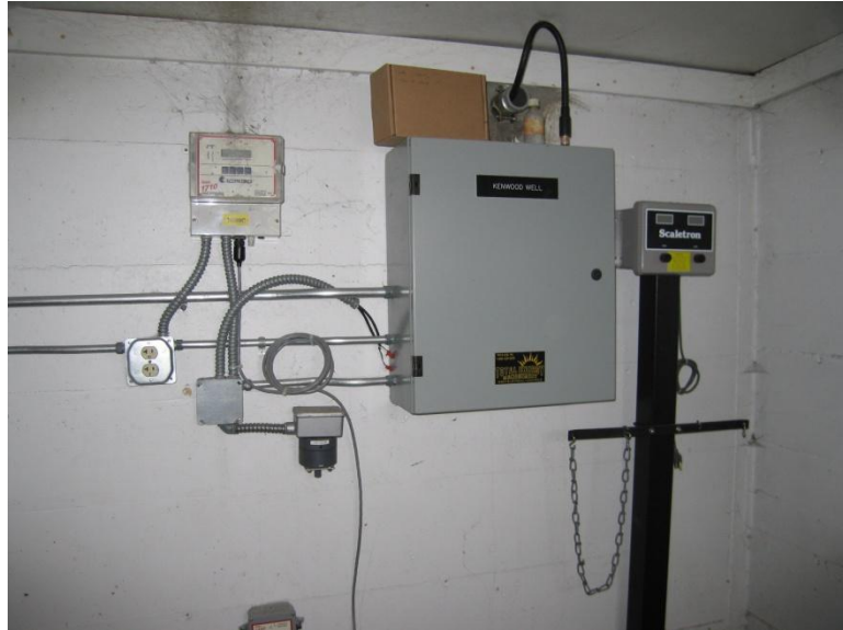
KENWOOD WELL CHLORINATION AND TELEMETRY PANEL
