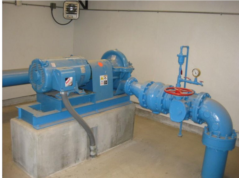
RIVERSIDE BOOSTER STATION PUMP & PIPING
