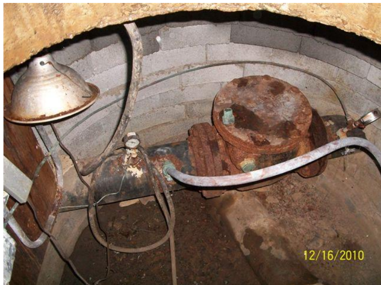
MONTVU BOOSTER CHECK & GAUGES
