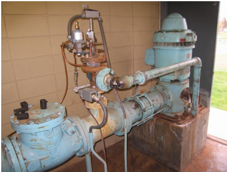
OKOMA WELL DISCHARGE PIPING
