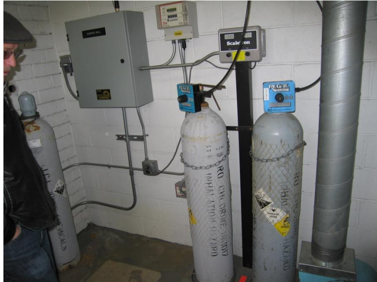
EASTSIDE WELL CHLORINATION EQUIPMENT
