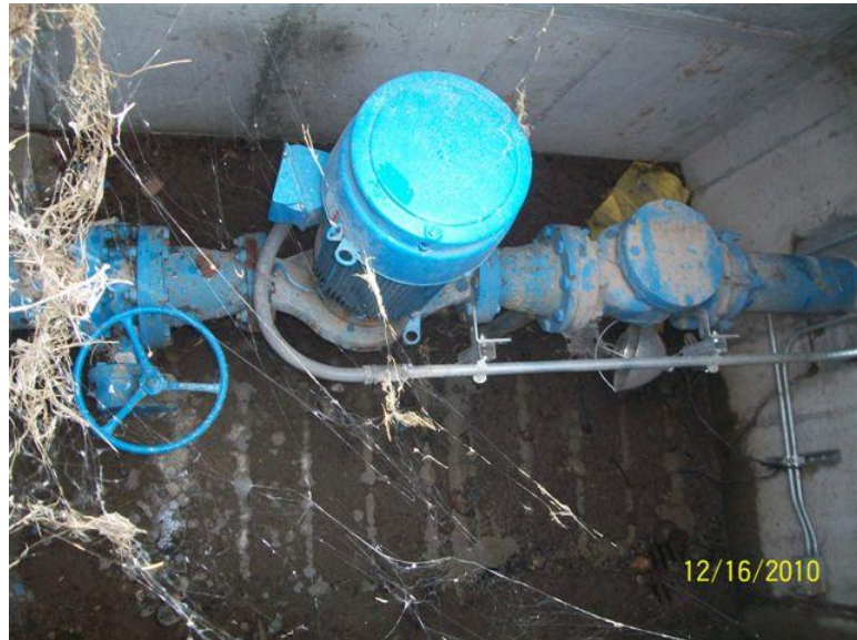
KOALA DRIVE BOOSTER PUMP & VALVES
