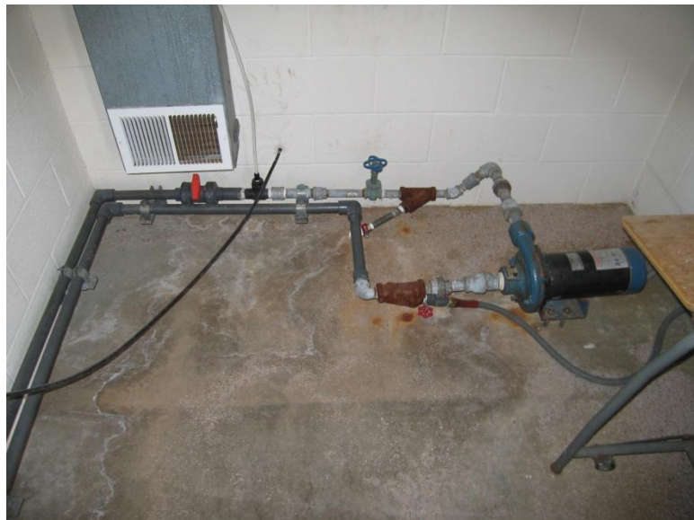
OWP WELL #2 CHLORINATION BOOSTER PUMP EQUIPMENT
