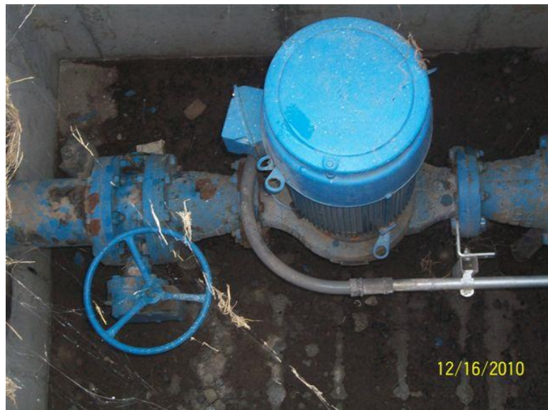
KOALA DRIVE BOOSTER PUMP & VALVES
