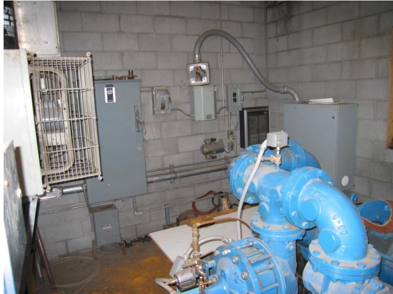
OWP WELL #2 DISCHARGE PIPING (WITH MOTOR AND PUMP REMOVED)
