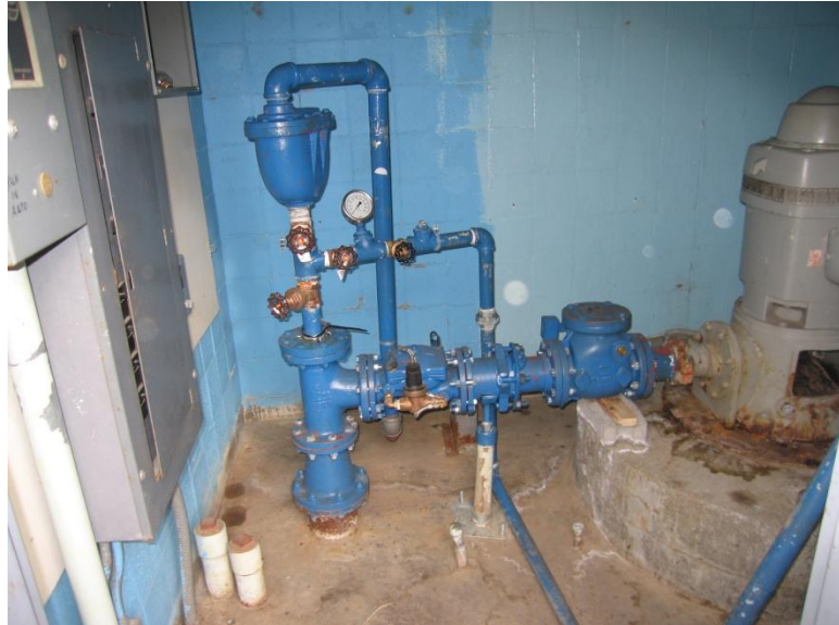
EAST OMAK PARK WELL DISCHARGE PIPING
