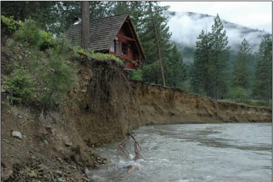
Figure 31) 2006 Landslide due to Flash Flooding in Methow River Valley.
