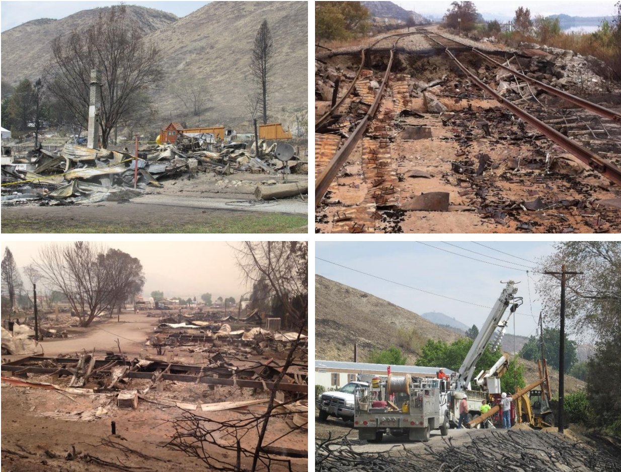
Figure 80) Damage to Pateros, WA as a result of the 2014 Carlton Complex fire.
