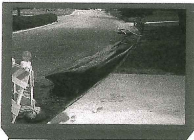
LVT filter bags are 75' long and 3' wide.
