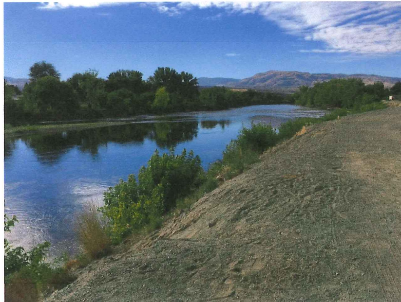
Figure 19. Okanogan River at downtown Omak viewed from levee.
